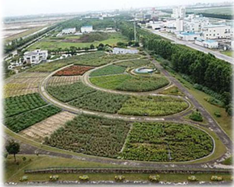
Vertical-flow soil filter on the constructed wetland, Changshu, China
